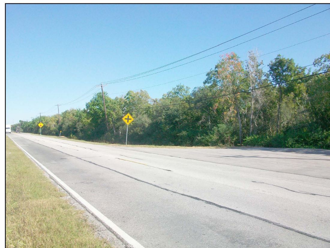
VIEW FACING NORTHWEST PROPERTY COR (TAKEN FROM TEXAS AVE)
