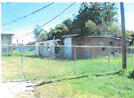
Abandoned commercial property fronting FM 1765
