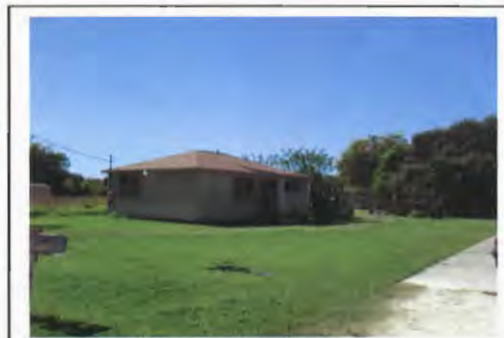
West side of Preston, mid-block
