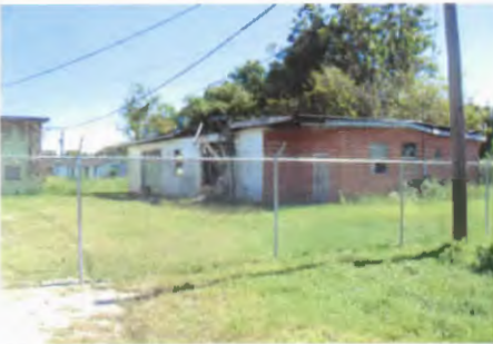
Abandoned commercial property fronting FM 1765
