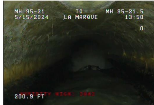
6, 00:07:15, 200.90ft Alignment Down, 20% changed
