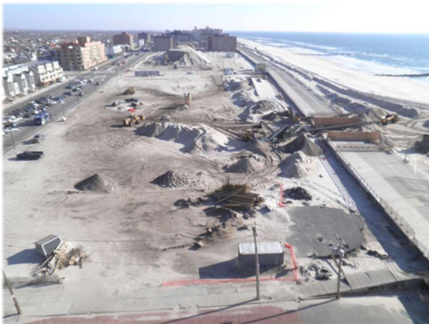
Sand Reclamation and Screening Site
