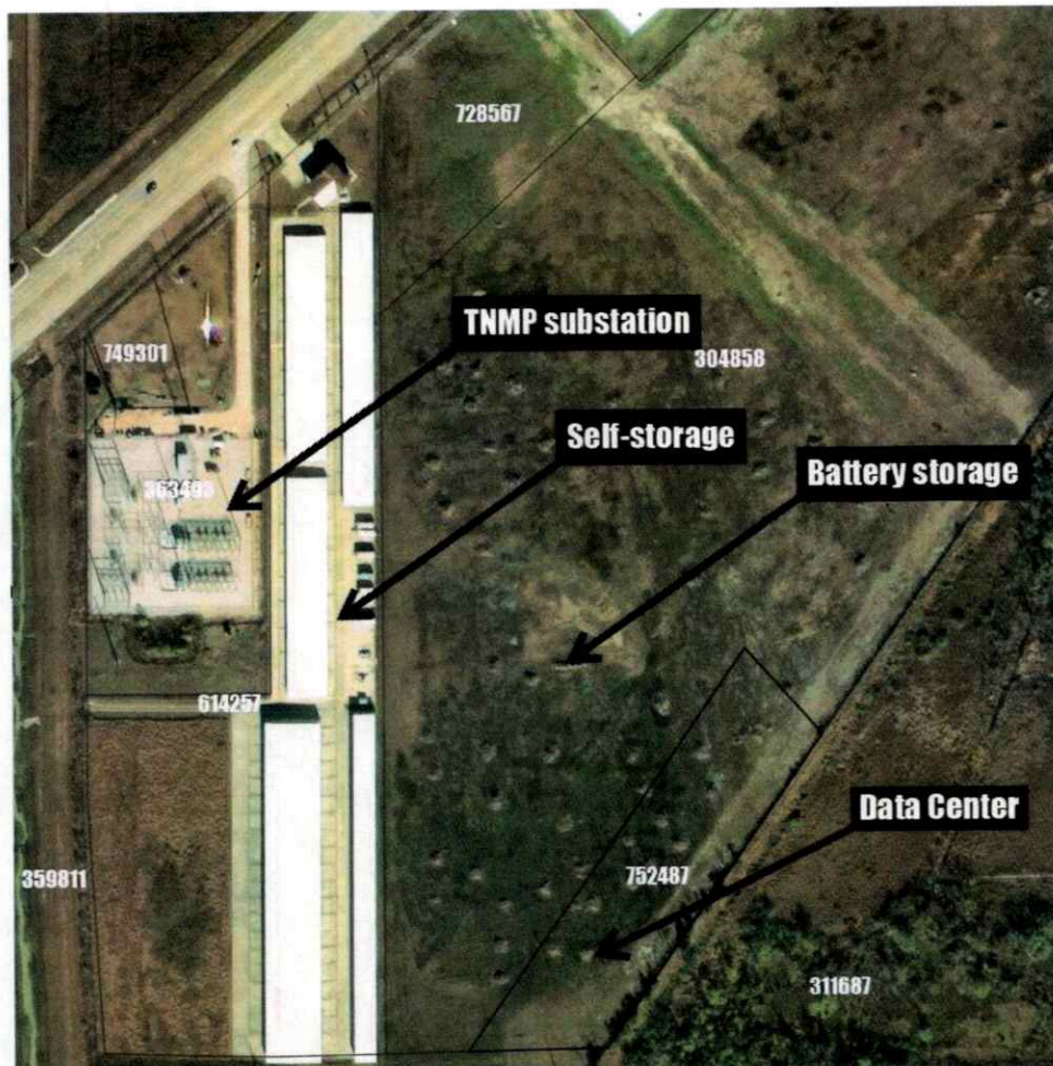
Data Center location
