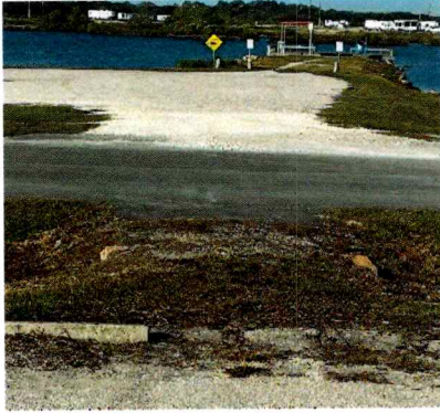
4th Crossing - Pavilion
