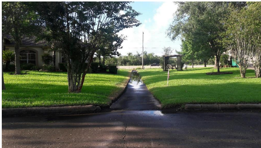
Concrete Swale No. 2
