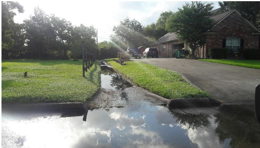
Concrete Swale No. 1
